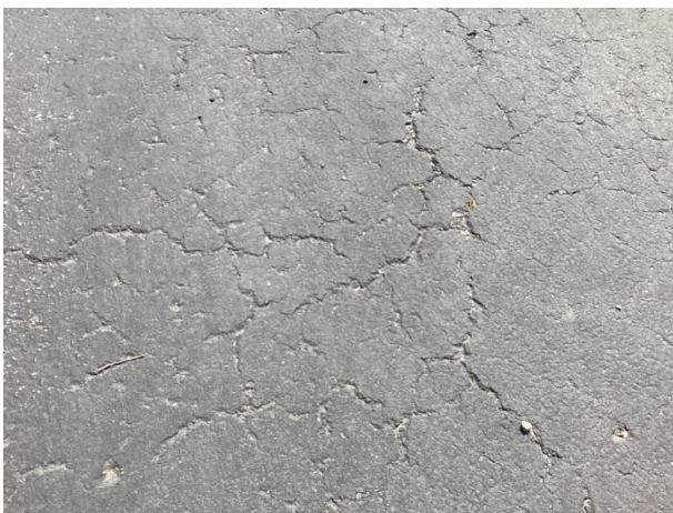
Alligator cracks
