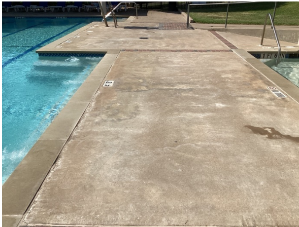
Concrete pool deck overview
