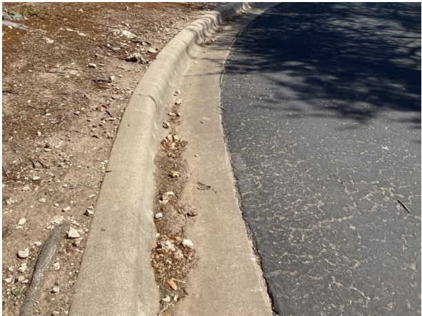
Concrete curb and gutter
