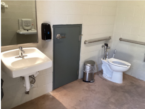
Rest room overview
