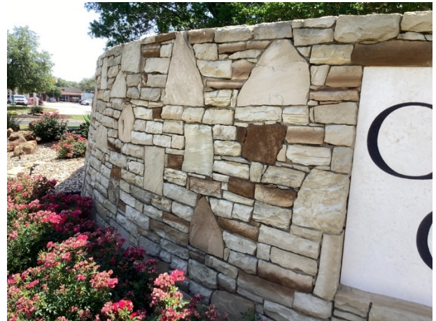
Masonry at monument
