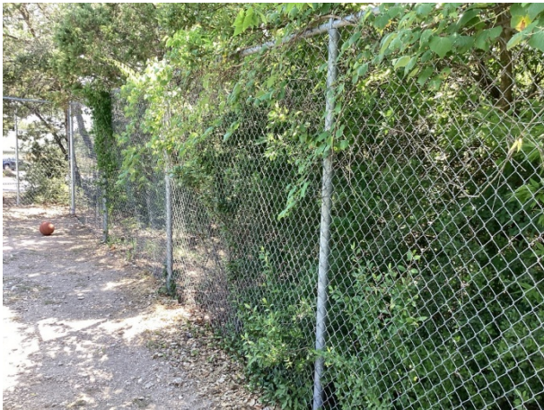
Chain link fence
