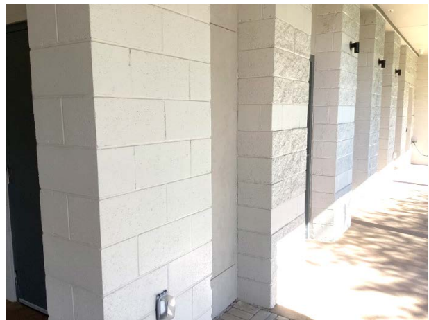
Painted CMU walls
