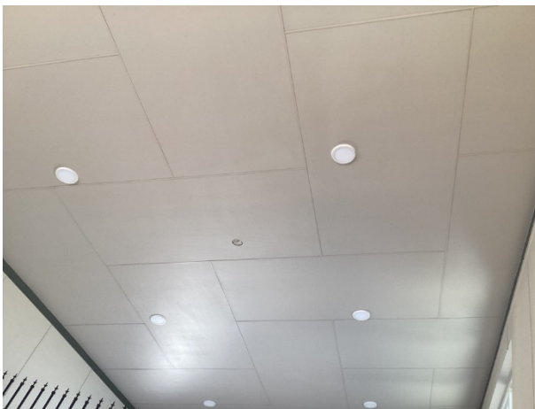
Paint finishes at soffit
