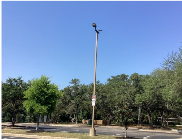
Light pole and fixture at parking area
