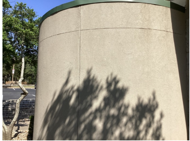
Stucco wall finishes
