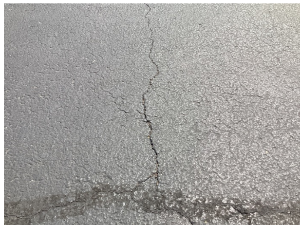
Pavement cracks
