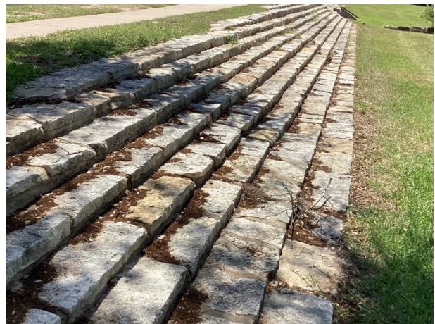
Mortar set masonry retaining wall
