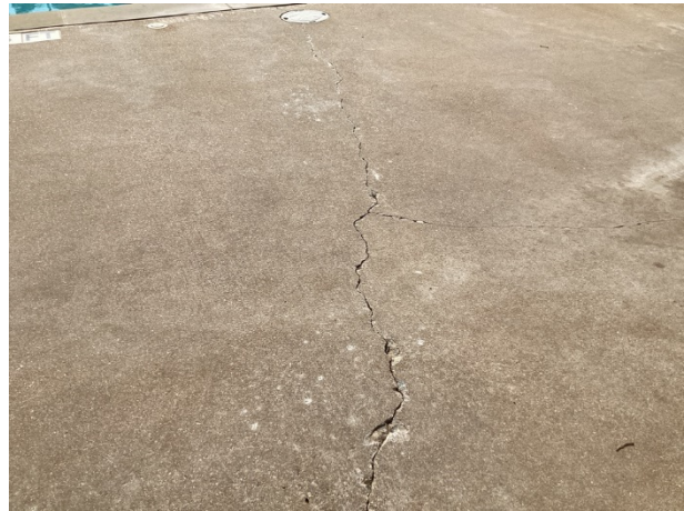
Concrete cracks
