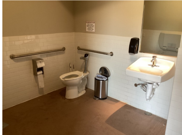
Rest room overview
