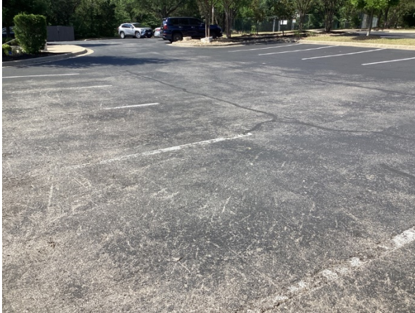
Asphalt pavement parking lot overview
