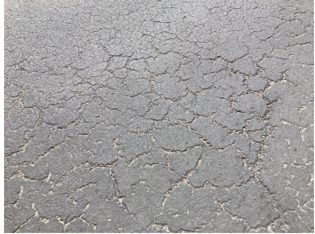
Alligator cracks
