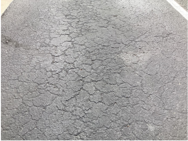
Alligator cracks
