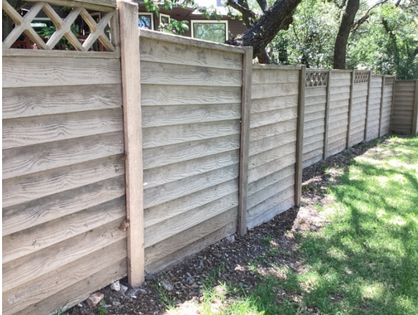
Concrete perimeter wall overview
