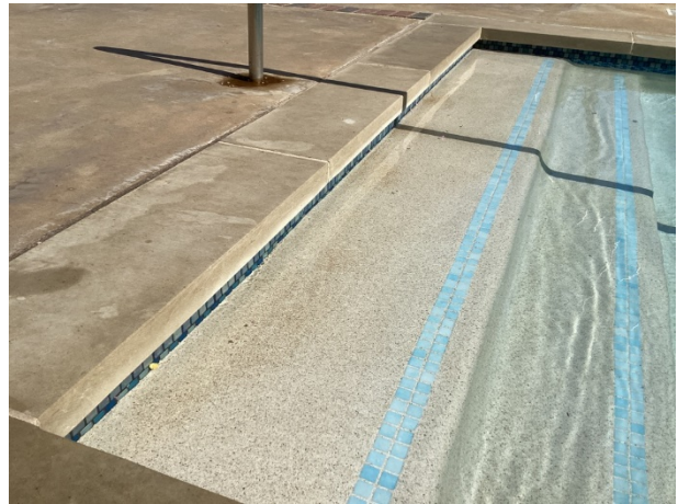
Pool plaster finish with tile and coping
