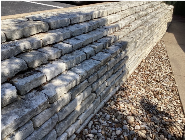
Masonry retaining wall at pool area
