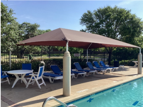
Shade structure overview
